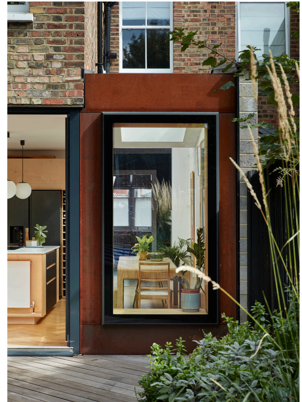
NOEL PARK, LONDON Extension and extensive renovation of a Victorian house in North London
